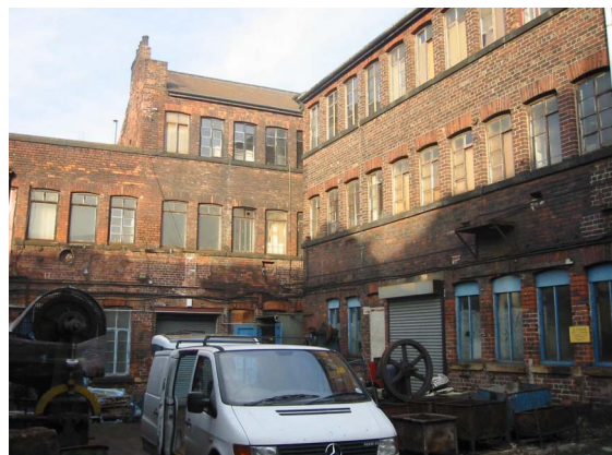
101. Internal courtyard of Portland Works (10), the buildings retaining many original windows.
