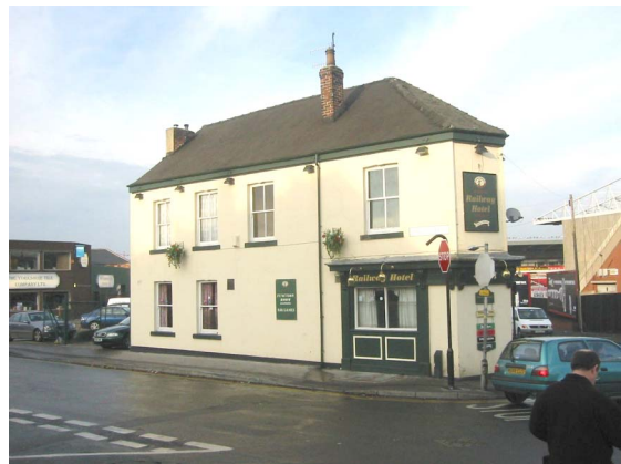
93. The Railway Hotel on the corner of Bramall Lane and Hill Street - defining the corner of the Conservation Area.
