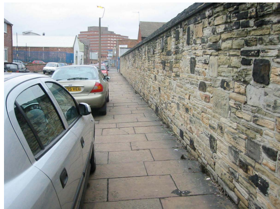
81. Surviving flagstone footpath on Arley Street.
