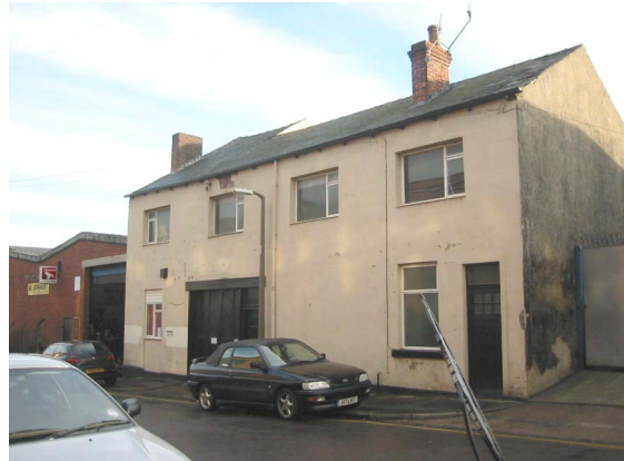
97. 84-90 Randall Street (11) - the brickwork is now rendered over and the windows replaced inappropriately.
